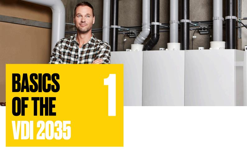
Cast iron boilers, voluminous designed pumps and welded piping was yesterday. Today's energy efficient heating systems require a good heating water quality: small and compact heat exchangers are more sensitive to hardness, efficient pumps and valves more sensitive to dirt, Aluminium alloys require a correct pH value, modern installation material call for a different view on corrosion protection (if any possible without chemicals).
